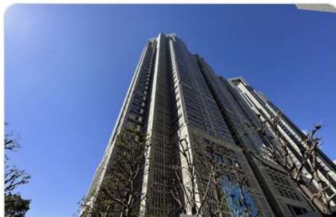
Tokyo Metropolitan Government Second Main Building 3rd floor
