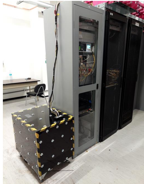
Laser interrogator in network shelter
